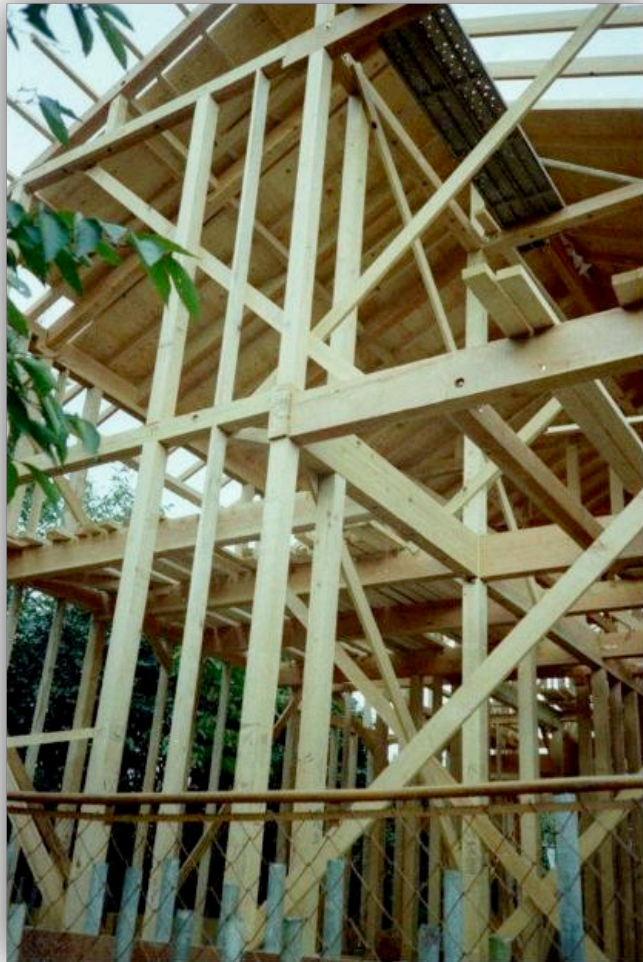
House under construction
