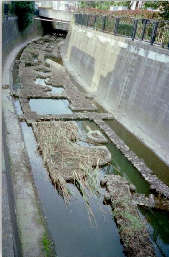
Canal structure at Mitakadai
